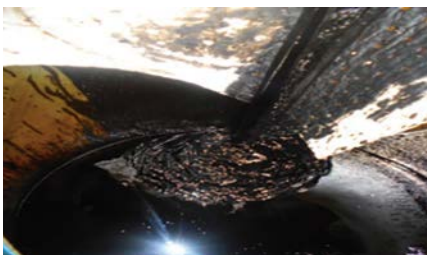
Hard Sludge in a FO tank – CHEM NEW YORK
